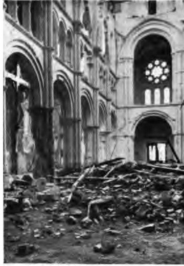
INTERIOR OF THE CHURCH OF ST. ANDRÉ
