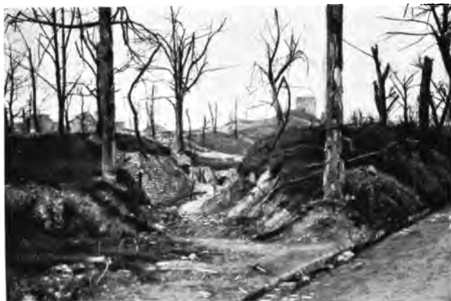
TRENCHES AND SHELTERS IN THE SQUARE ST. NICAISE
