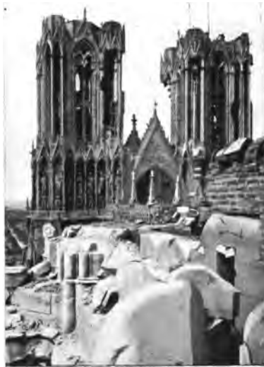
ROOF OF THE NAVE IN 1919
