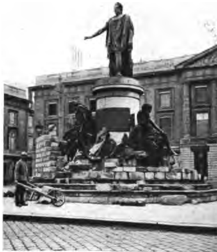
STATUE OF LOUIS XV., PLACE ROYALE, WITH PARTIALLY BUILT PROTECTING WALL OF MASONRY
