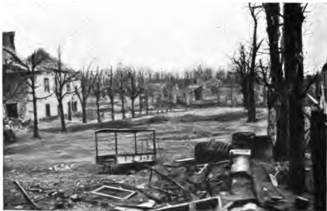
THE "PLACE DE LA MAIRIE" AT SILLERY (1918)
