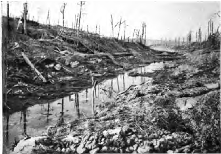
THE AISNE CANAL AT THE "CAVALIERS DE COURCY"
