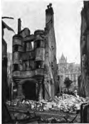
DOOR OF THE CHAPTER-HOUSE COURTYARD
