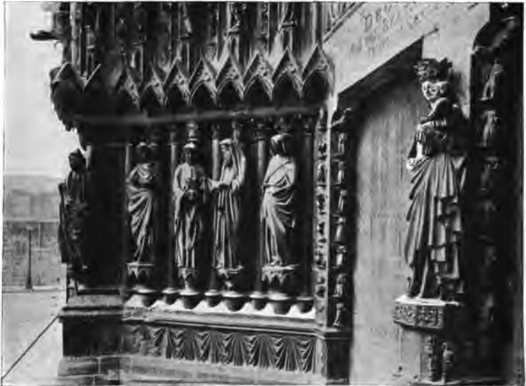
LEFT-HAND SPLAYING AND LINTEL OF THE CENTRAL DOOR ( Cliché LL. )
