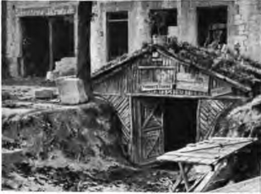
ENTRANCE TO "POMMERN TUNNEL" AT WITRY-LES-REIMS
