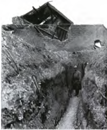
COMMUNICATING TRENCH AT JOUISSANCE FARM (1915)
