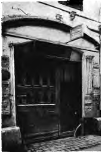
14TH CENTURY DOORWAY, 22 RUE DE TAMBOUR
