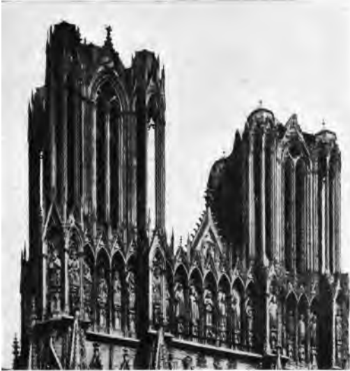
SECOND STOREY AND UPPER STOREY OF THE TOWERS
