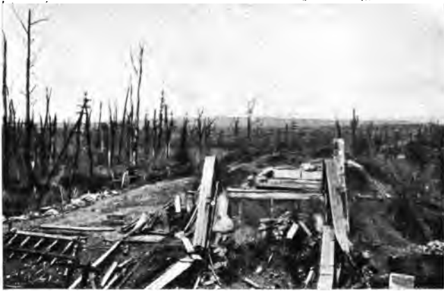
DESTROYED BRIDGE OVER THE CANAL, NEAR LE GODAT
