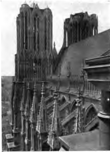
ROOF OF THE NAVE IN 1914
