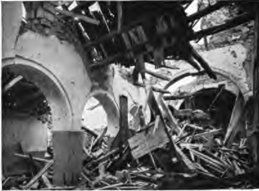
THE INSIDE OF ORMES CHURCH
